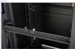
4-point horizontal stiffeners
